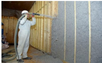
FIGURE 2 EXAMPLE OF HEMPCRETE BLOW IN
