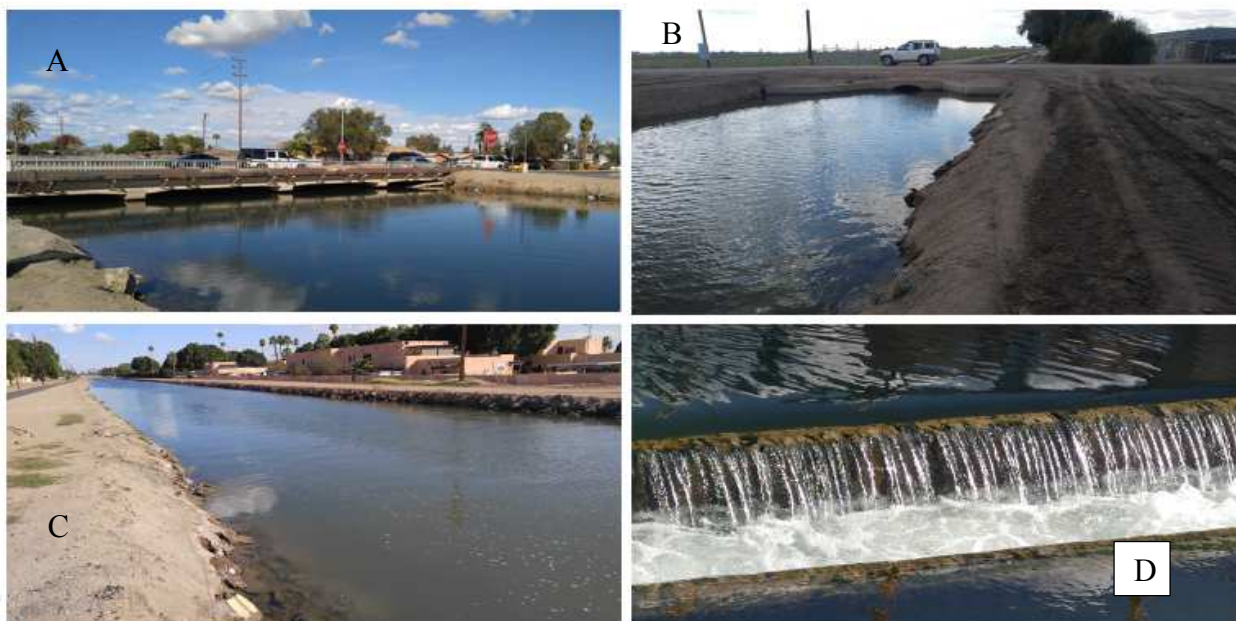
Figure 3: Images of Irrigation canals: Image A shows an irrigation canal in an urban area with a bridge and traffic. It is very wide and is unlined and is surrounded by neighborhoods and has ducks that reside under the bridge. There is also trash in the canal. Image B shows a suburban unlined irrigation canal; the canal is large and is near some houses and warehouses on the right side and fields on the left side. Image C shows a wide unlined urban irrigation canal near apartments, houses, businesses, and a bike path. The water in image C is a brownish/turbid color; the water flow is slow near the canal banks. Image D shows a mixing station in an Irrigation canal, the water here is moving fast.
