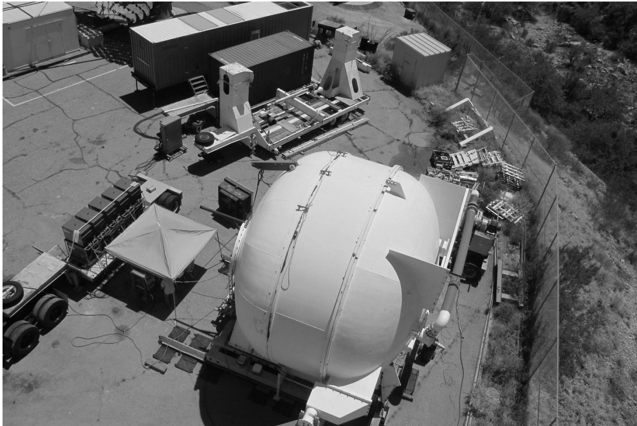
Figure 3 – MMTO full-scale coating test facility. There is enough electrical power available to run the vacuum pumps, but a mobile generator (in the long shipping container near the top of the image) was rented to provide power to the welders.
