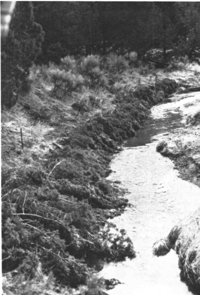
*Vegetative riprap made by suspending and securing cut juniper against an eroding streambank.*
