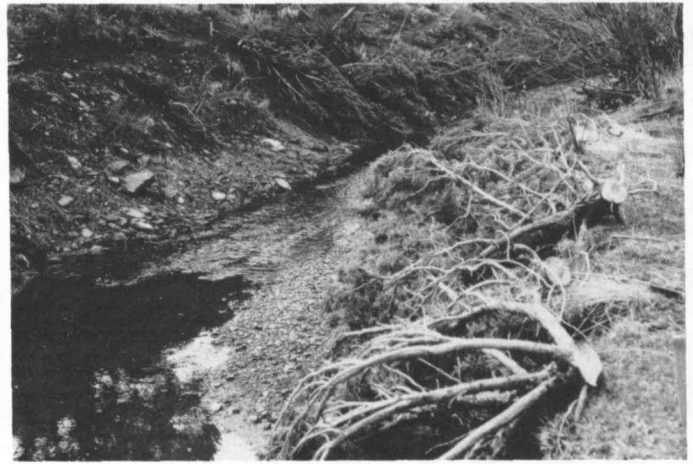
Juniper Creek showing cut juniper trees cabled along the stream for bank stabilization.
