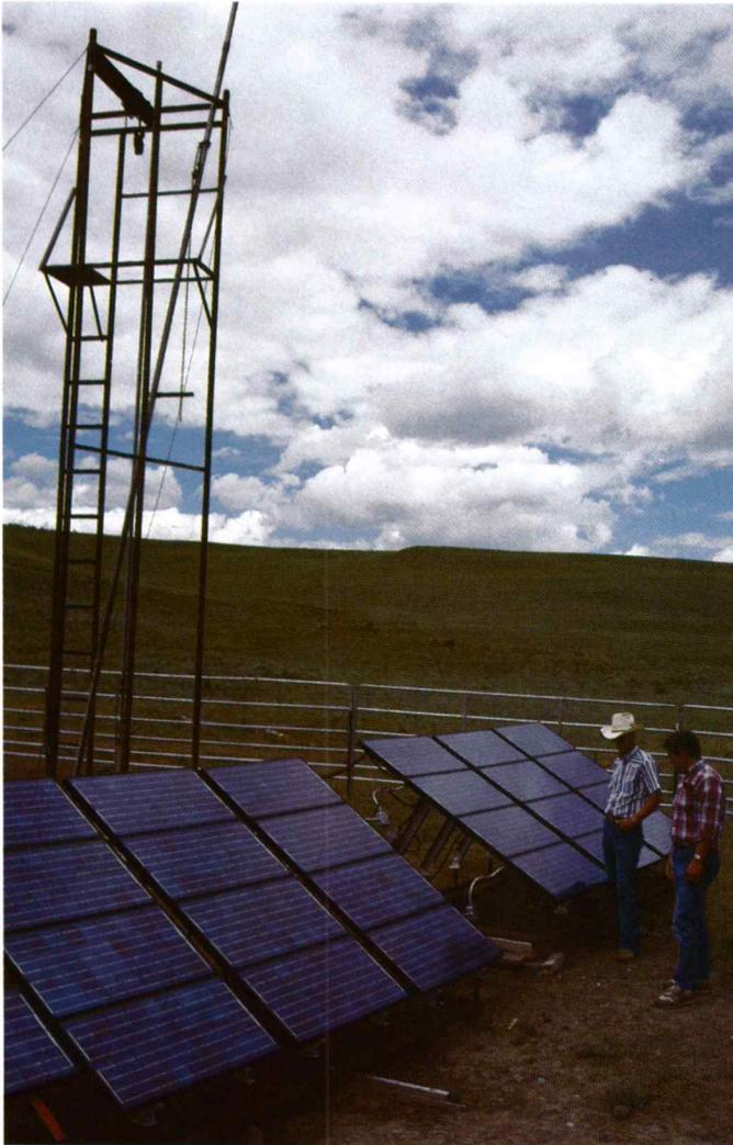
SCS Conservationists Burl Boren and John Valentine inspect solar powered water system which can supply 40,000 gallons per day.
