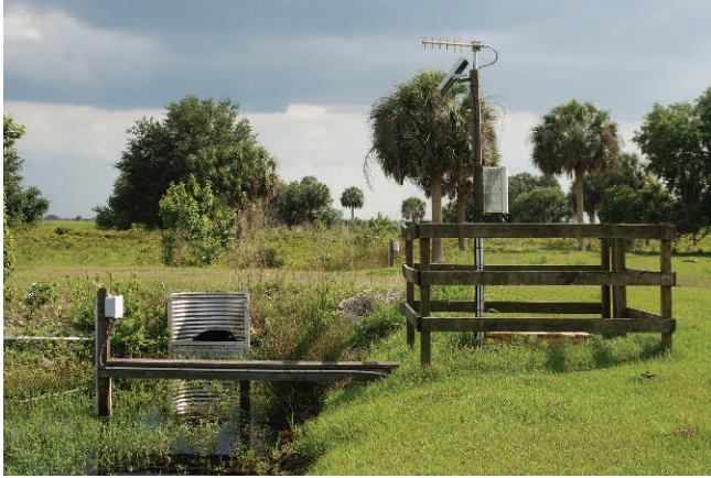
Figure 6. One example of a NE-PES monitoring site. Water stage is recorded every 15 minutes by a pressure transducer and the data is stored in a datalogger in a waterproof box mounted to the wooden post. A solar panel powers the station. A rain tipping bucket is at a nearby monitoring station. Photo courtesy of Elizabeth Boughton.
