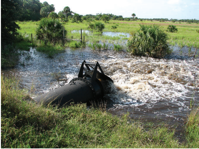
Figure 2. Water is pumped into a 2,500 acre marsh from a regional canal where nutrients are sequestered by natural processes. Photo courtesy of Earl Keel.
