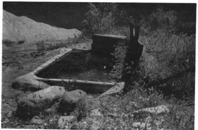
Fig. 2. A working sand dam on the Tonto National Forest near Phoenix, Arizona. Water is collected in pipes behind the dam (top photo). Water is made available to animals in a trough fitted with a mechanical float valve (bottom photo). Photo dates May 3, 1979.
