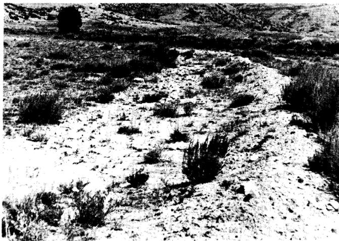
**Fig. 1.** Roadways had all been made by a grader or bulldozer passing over the site to clear off brush and smooth off surface irregularities. Plant debris and surface soils were windrowed into a berm at roadside. There had been no attempt to form gutters or elevate roadbeds. Plant life persisted in the center of all roads sampled.
