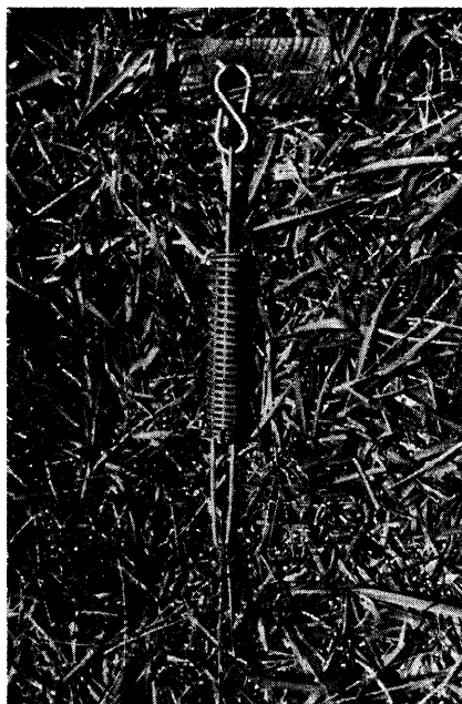
FIG. 2. Spring installed and adjusted to about 25-lb tension.
