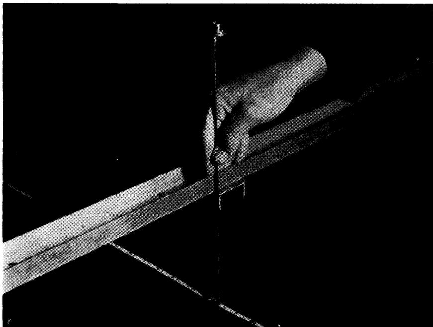
FIGURE 2. Using the 3/4-inch loop to plumb the frame over the tape mark of a frame position when the tape lies below the adjustable height of the frame.
