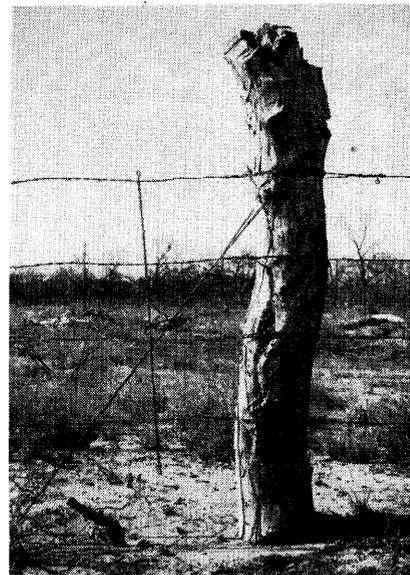
Support posts are placed every ¼ mile. The support consists of a deadman anchor set 2 feet in the ground and attached to the post with No. 9 smooth wire. The twisted wire stays, as shown, are placed every 10 feet to keep the animals from forcing the wires apart.
