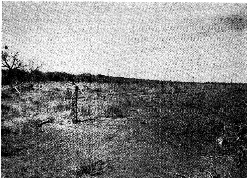
Posts in the suspension fence are spaced 100 feet apart. Line posts are 7 feet long, 6 inches at the tops, and are put 2½ feet in the ground. The fence is anchored every ¼ mile, and the strands are held apart by 40-inch twisted wire stays placed every 10 feet. The fence has a spring action between posts and has been very effective in holding animals. The approximate cost of construction in south Texas has been \$250 per mile.
