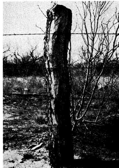
Line post in the suspension fence. The 12½ gauge wire is fastened to the post with a ¾-inch galvanized plate, 1 inch long, held in place with two eight-penny nails driven through holes punched in the plate. Staples are not satisfactory for holding the wire to the line posts in this type of fence.
