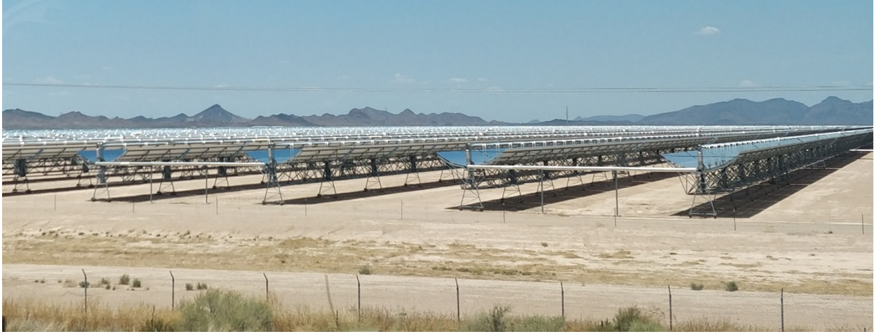
FIG. 2. Photograph of the Solana CSP system near Gila Bend, AZ, USA.
