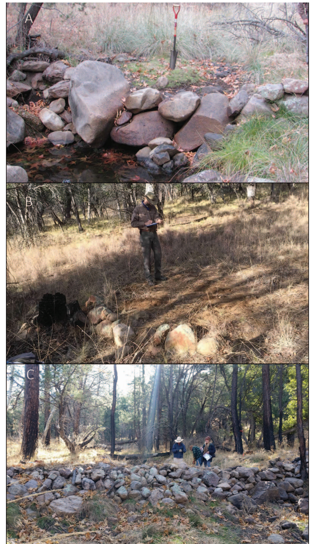
Figure 2. Examples of erosion control structures (ECS) used in the study. Location names: (A) Middle LBSO, (B) Hillslope LBSO, and (C) Middle HBSN.
