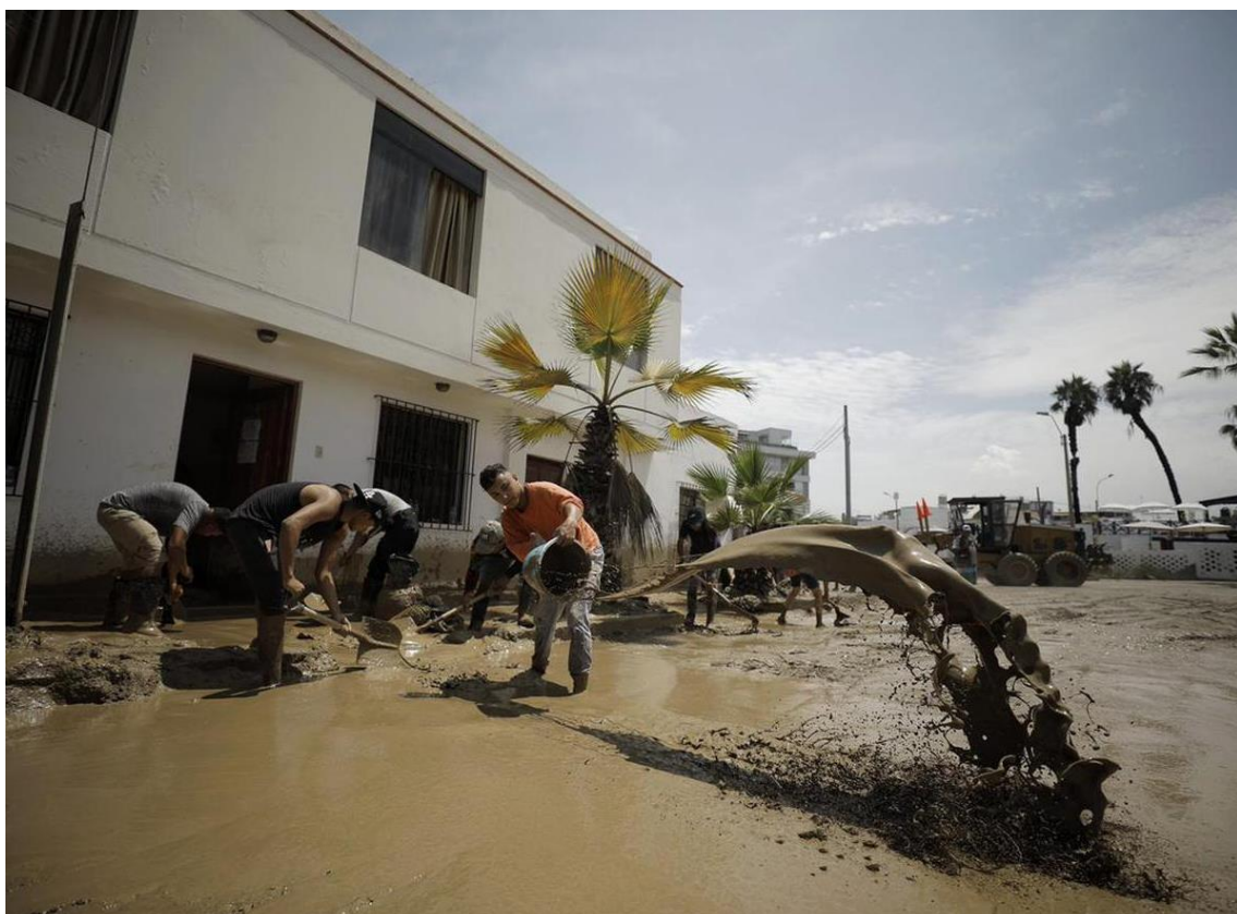
Figure 1. Photograph of residents cleaning up after the March 2023 Punta Hermosa landslides. Retrieved from Alonzo, 2023.
