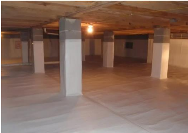
Figure 9-Encapsulated Crawlspace
