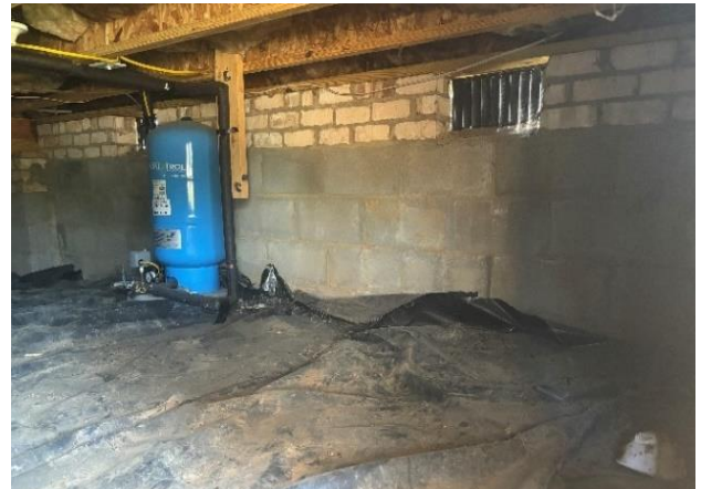
Figure 10- Vented Crawlspace
