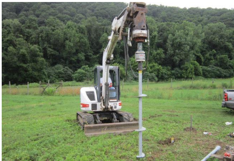
Figure 1. Helical pier being installed.
