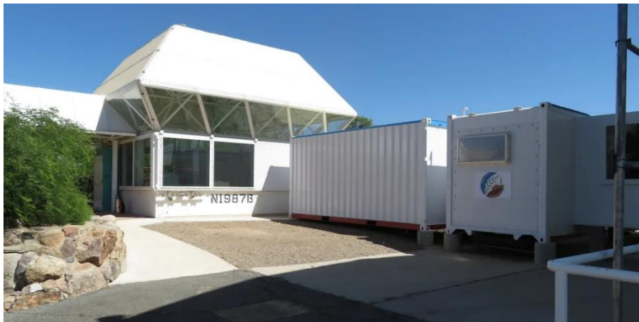
Figure 1 The SAM Test Module made of steel and glass (design wouldn't be used in space), the perpendicular 20ft container engineering/medical bay, then 40ft crew quarter container and air lock to the right
