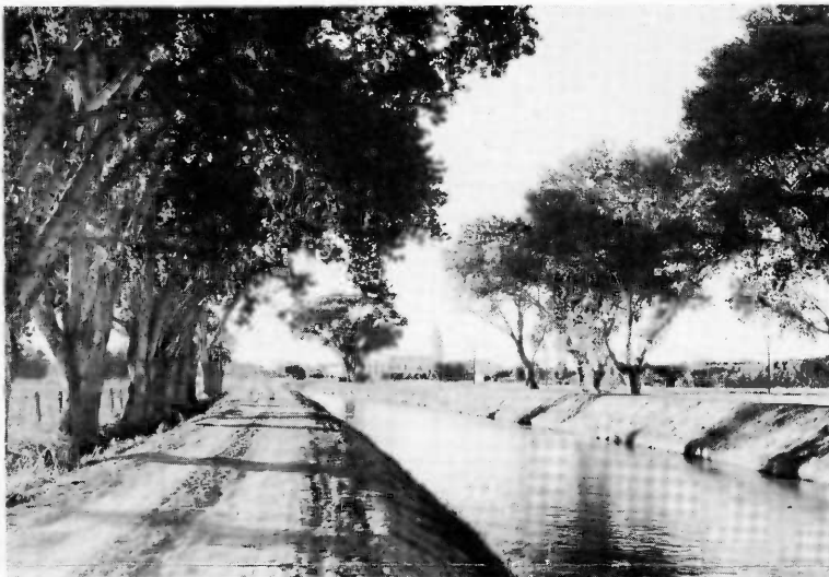
GRAND CANAL. SALT RIVER PROJECT
