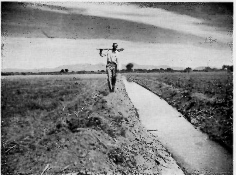
Straight ditches like this may be cleaned by machinery, saving much time and labor.
